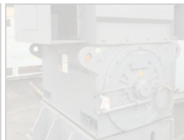
HITACHI INDUCTION MOTOR 1000 HP; 710 RPM Type: EFOA-KK; Frame: 450 LM 60 hertz; 1000 Volt
